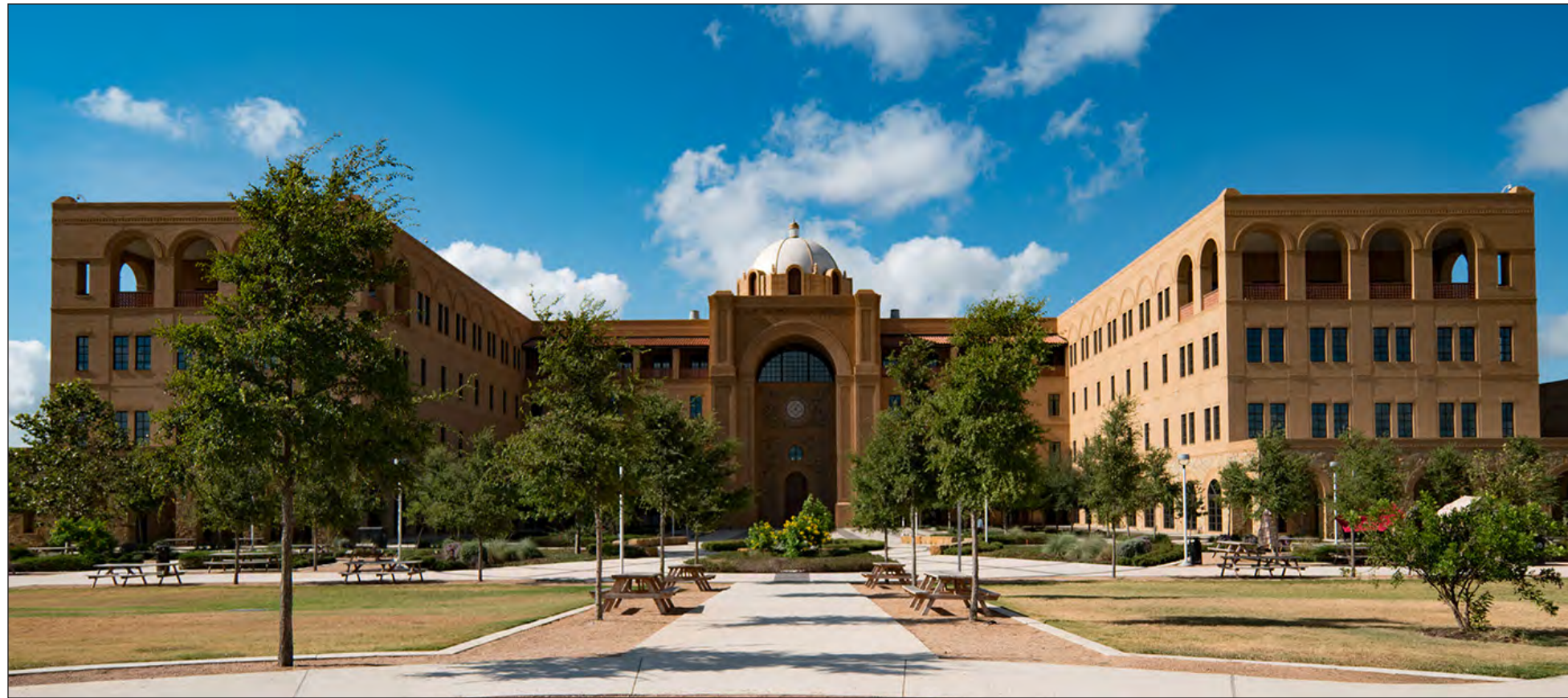
Texas A&M University-San Antonio Central Academic Building
